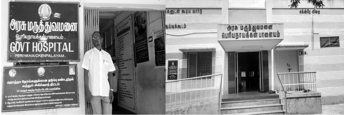
Fig. 6 : Periyanaickenpalayam Government Hospital (GH) Old & New Buildings
